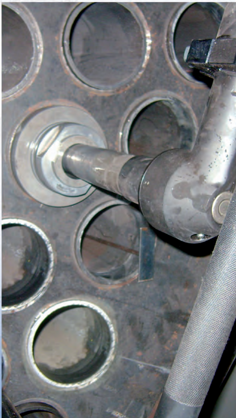
Expansion detail with Masterol 90 on boiler
